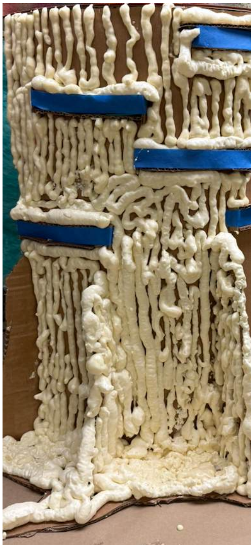
Figure 37. Expanding foam right after being applied
